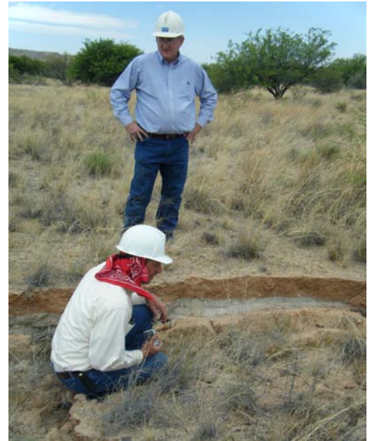
Several inches of dark colored cap material cover lighter colored tailing at Pima 6 Tailing. A subsidence feature is examined by Dan Robinett (contractor) and Al Richins (ASARCO).
